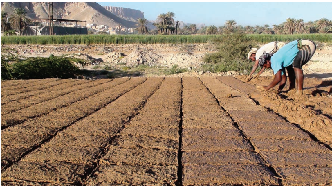
Preserving traditional building materials – Shibam, Hadhramaut
