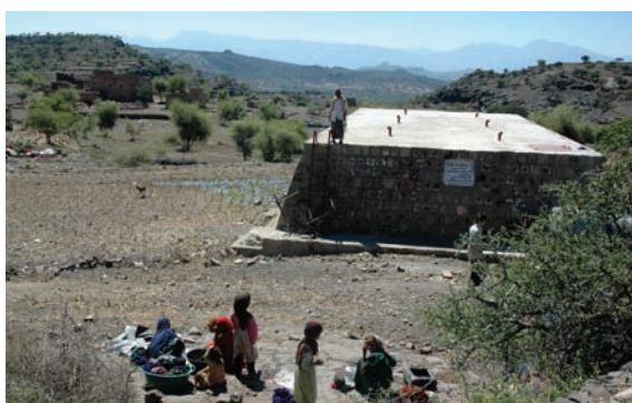
Rainwater harvesting tank - Isam Warafi'a, Asaweda, Taiz
