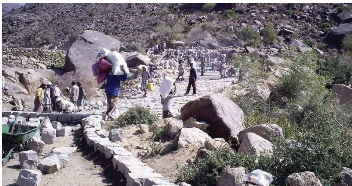
Labor-intensive works – Wesab, Dhamar
