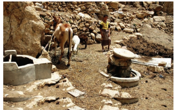
Biogas unit—Bora', Al-Hudaidah
