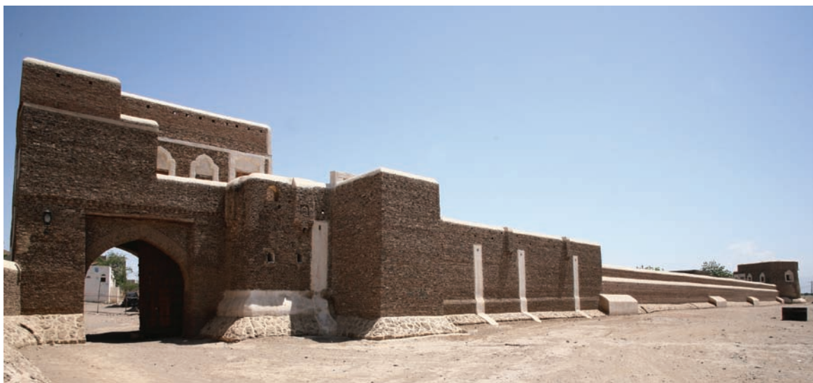
Bab Alqurtub Gate renovated- Zabid, Al-Hudaidah
